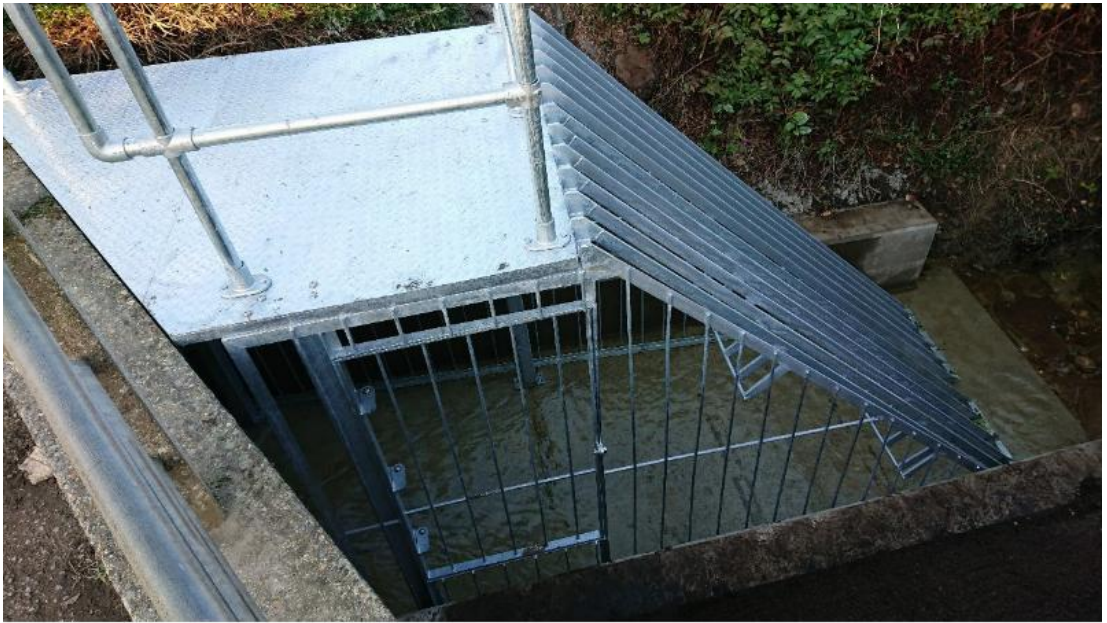
New Trash Screen at Mill Lane
