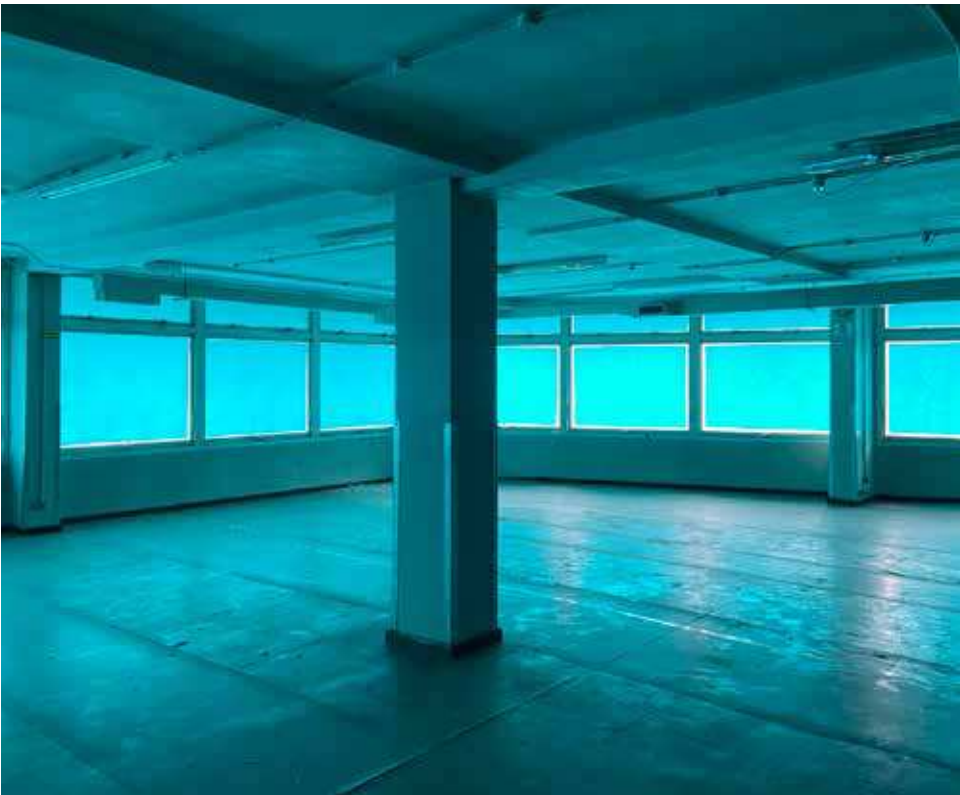
Existing first floor - exposed structural frame
