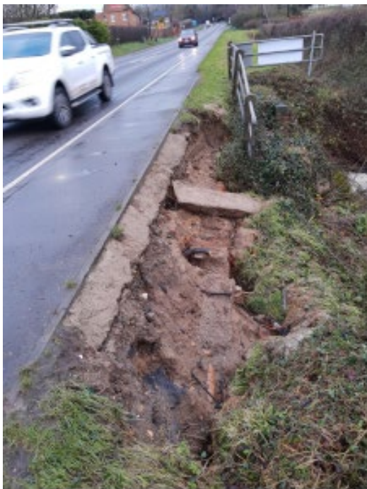
Figure 4: Section of bank slippage at A140 Swainsthorpe
