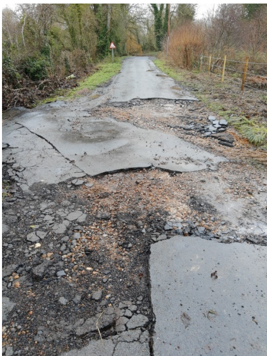
Figure 5: Section of road washed away by flood water at Newton Flotman – Mill Lane.
