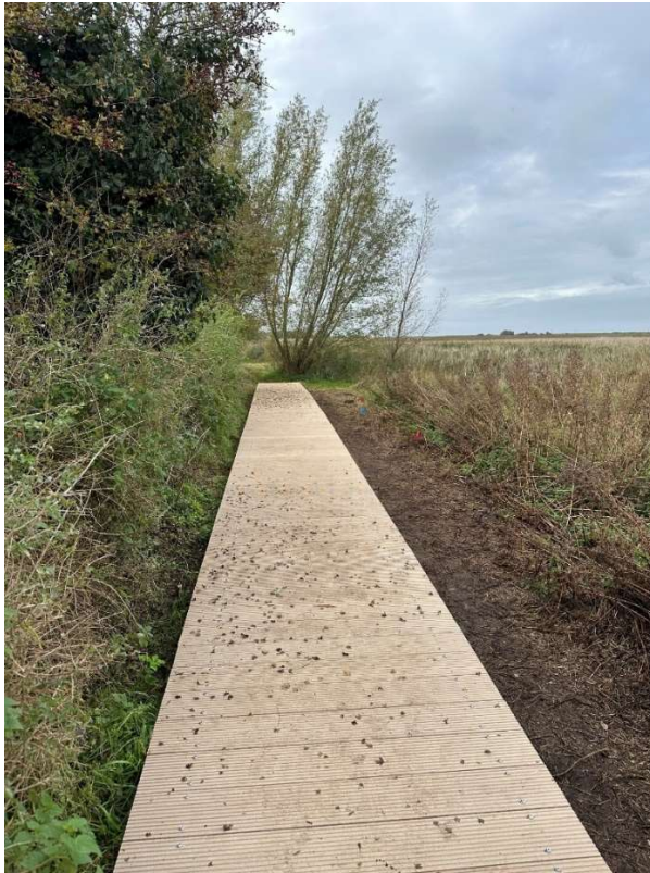
New GRP decking planks (bump strips to sides and passing places still to be installed)
