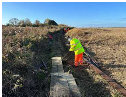
Construction (all hand/power tools only) Removal of timber boardwalk (all by hand. No machinery to assist removal)
