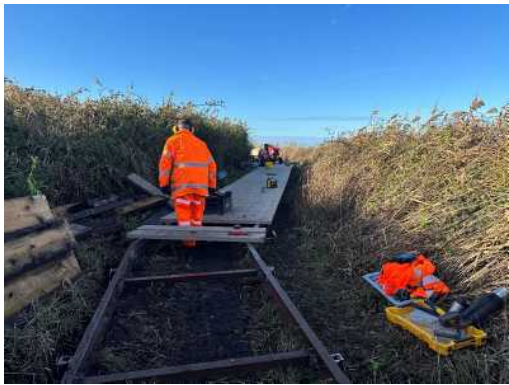
Construction (all hand/power tools only) Removal of timber boardwalk (all by hand. No machinery to assist removal)
