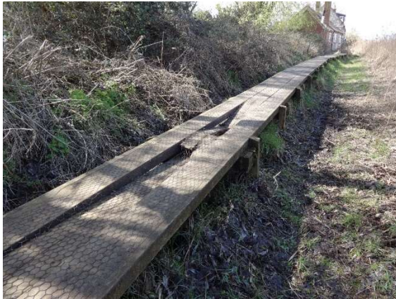
Condition of original timber boardwalk to be replaced.
