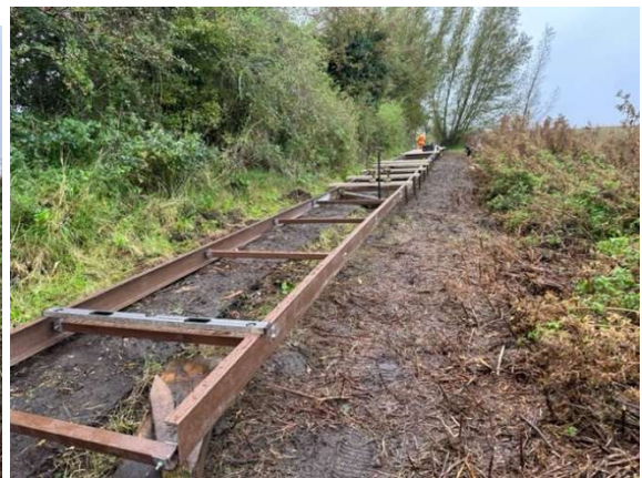
Installing new GRP substructure
