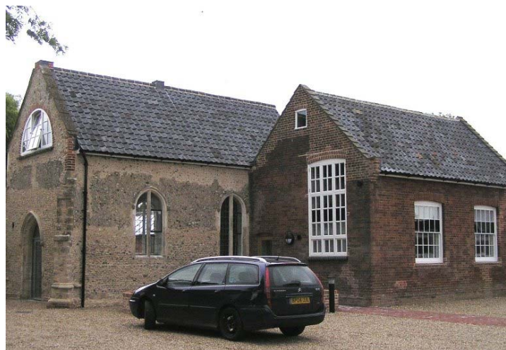
Pennoyer's School, Pulham St Mary, before and after restoration.
