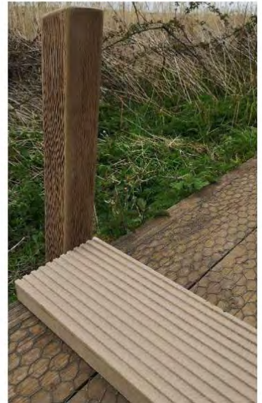
Contrasting wood-effect handrail.
