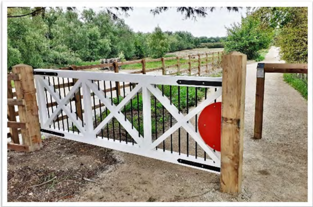
Station Road - After
