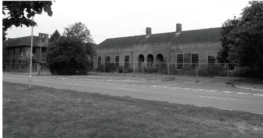
B - Existing front elevation of the Officers' Mess.
