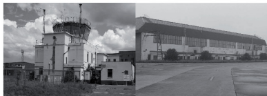
③ Station Control Tower Locally Listed ④ Hanger Locally Listed
