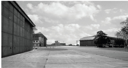
A - Existing technical area.
