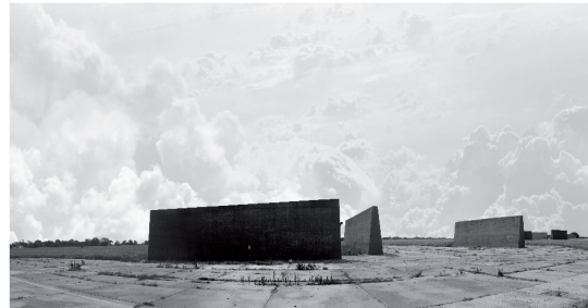
F - Existing Cold War Revetments
