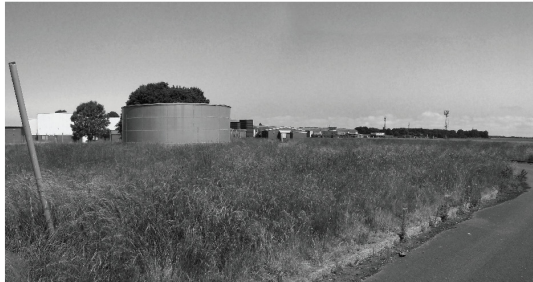
D - Existing storage tank at entrance to Piggyery lane.
