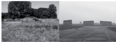
① WW2 Protected Dispersal Point Ancient Monument ② Blast Walls Ancient Monument
