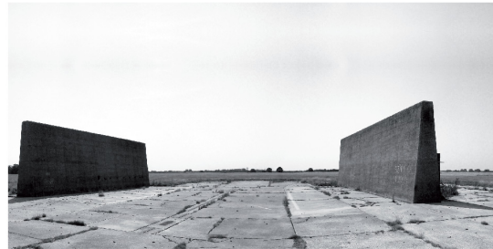
E - Existing Cold War Revetments.
