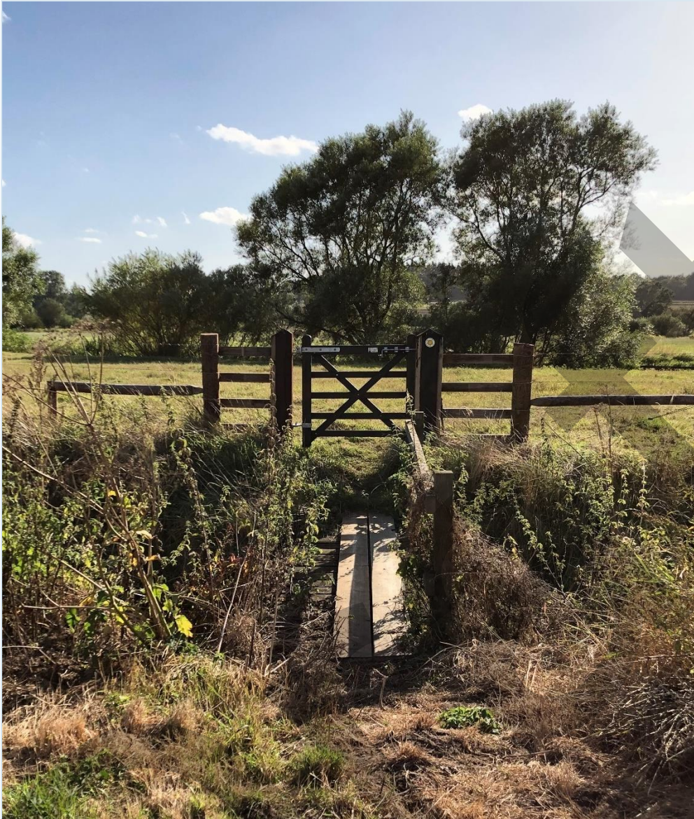
Figure 2-33 - Site 7, Narrow bridge across watercourse
