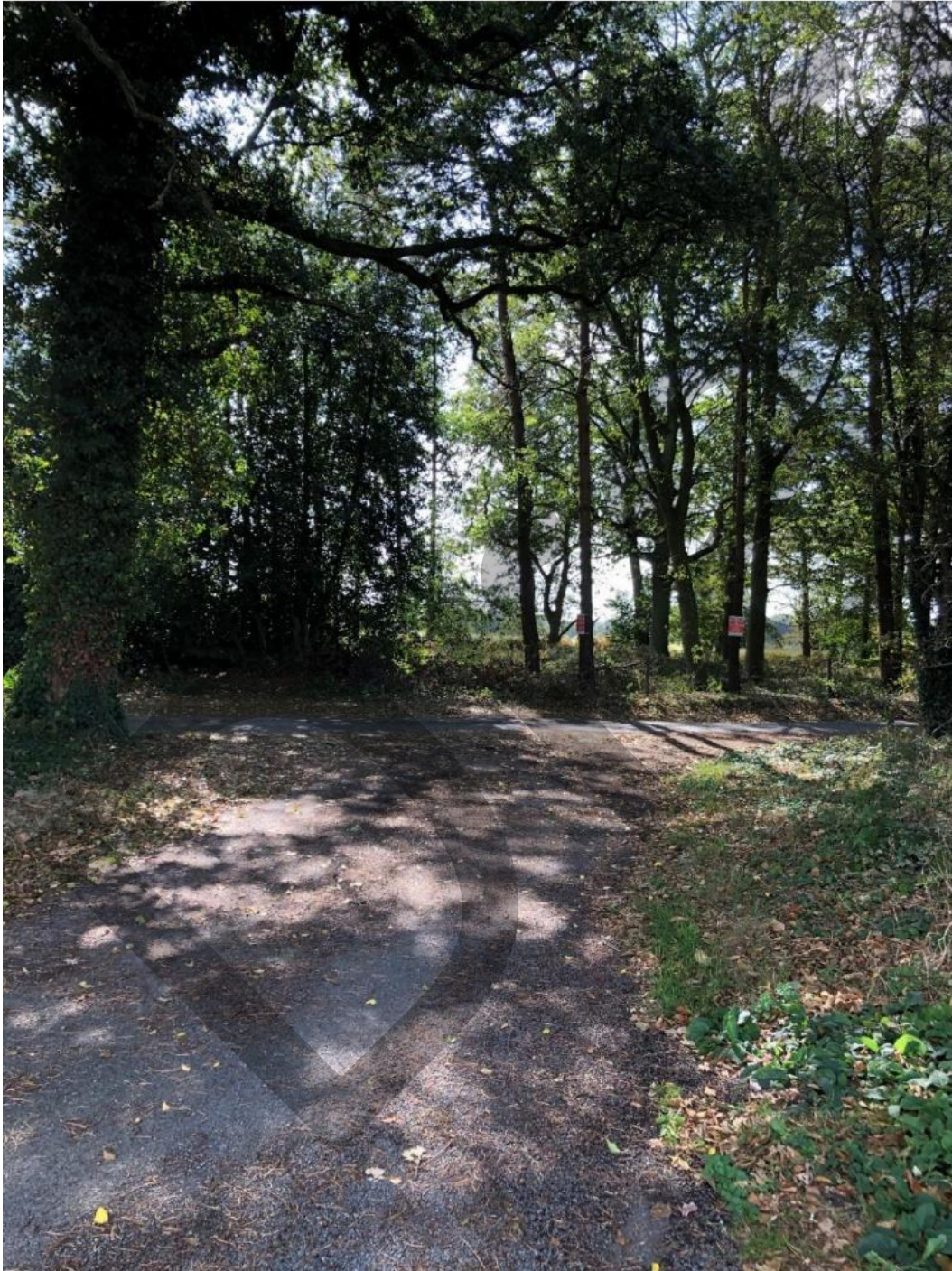
Figure 2-19 – Site 2, Priority junction from the Broadway (east), onto Breck Road
