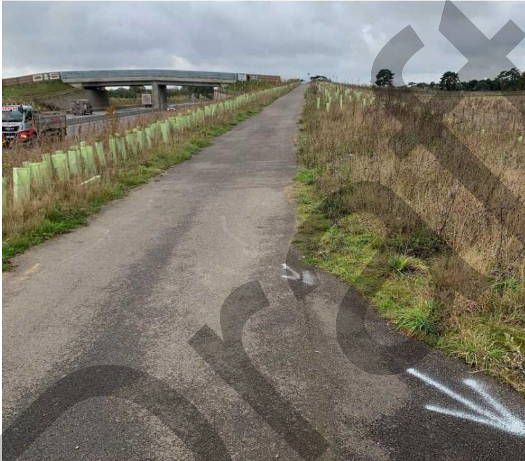
Figure 2-53 – Marriott's Way bridge, access from Furze Lane
