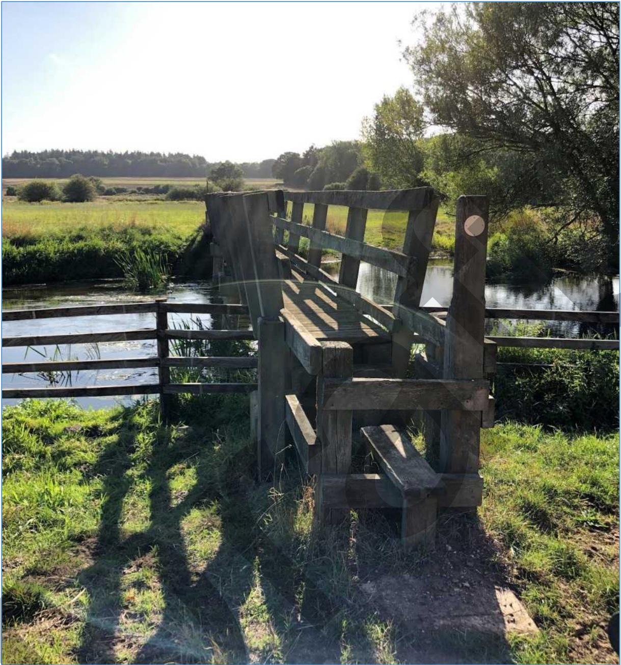
Figure 2-35 - Site 7, Footbridge across the River Wensum
