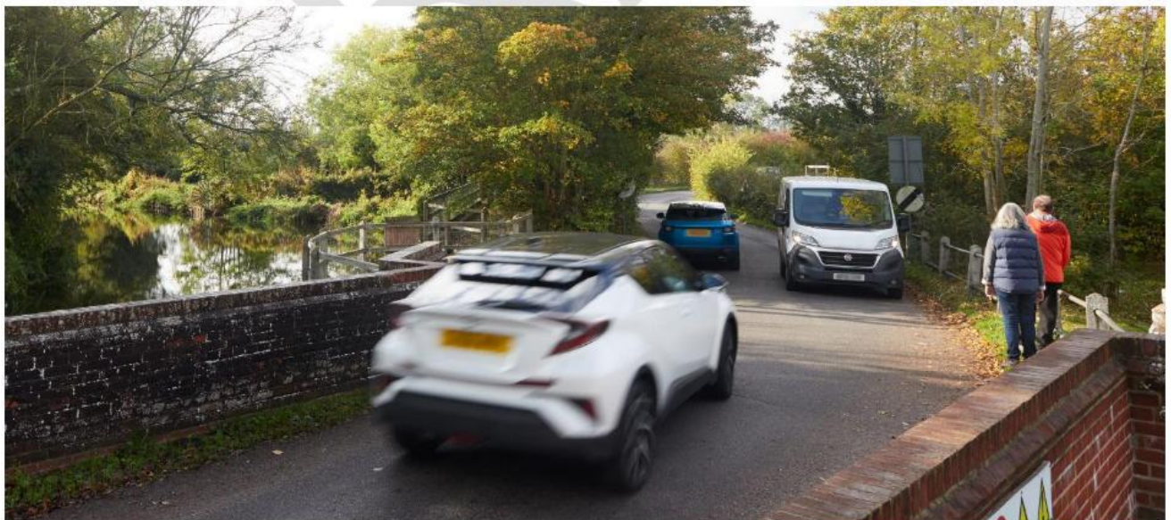
Figure 2-15 - Costessey Lane Bridge
