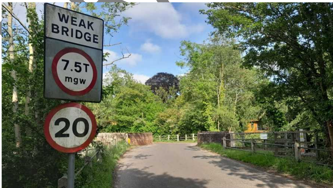
Figure 2-10 Costessey Mill Bridge, Costessey Lane
