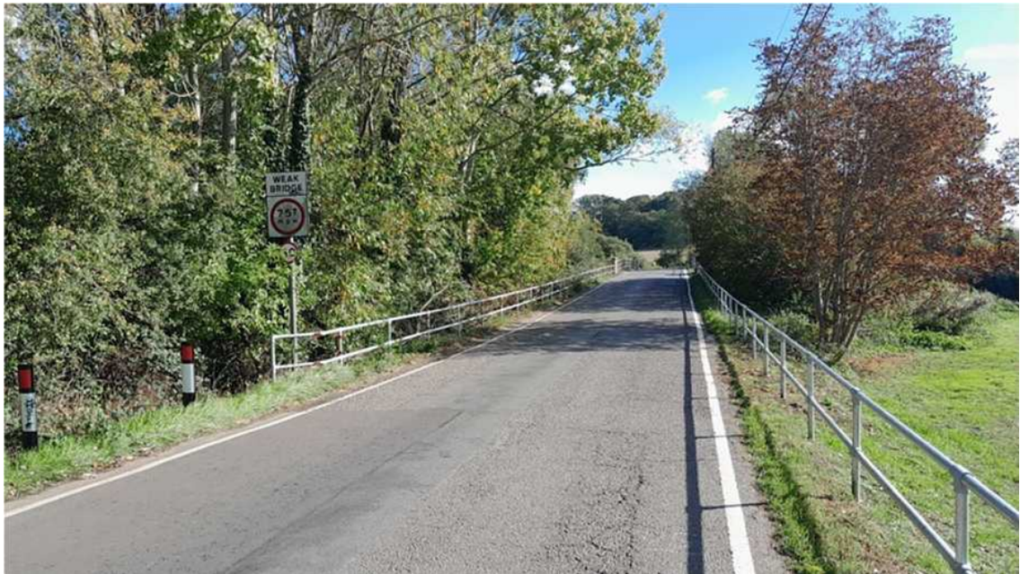
Figure 2-11 Ringland Road Bridge
