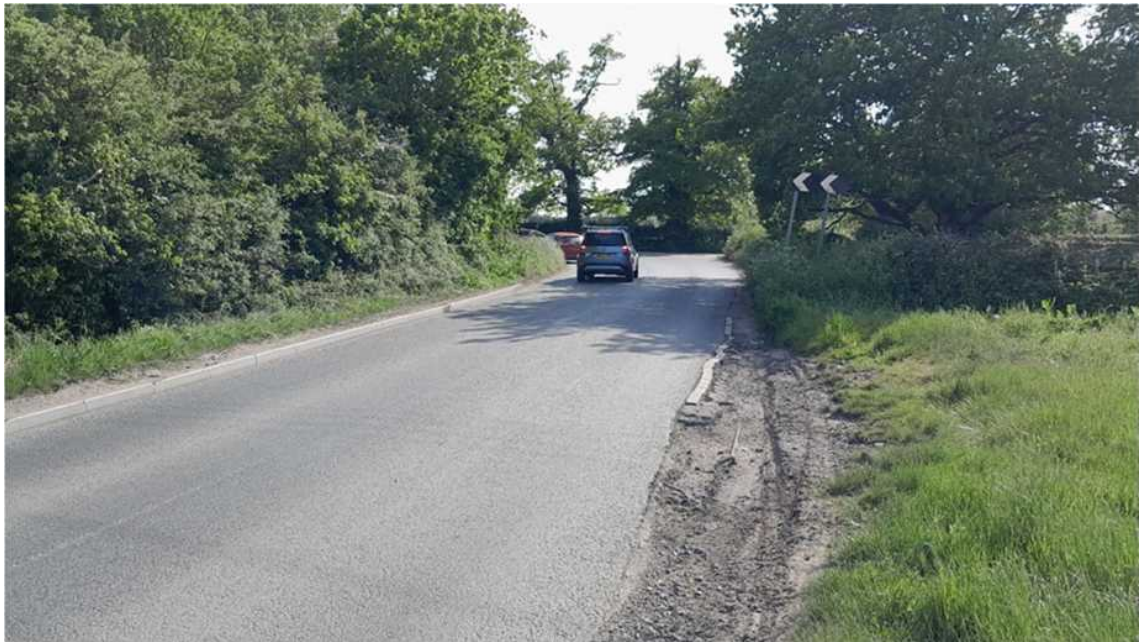
Figure 2-7 B1535 Tight Bend at Rectory Road
