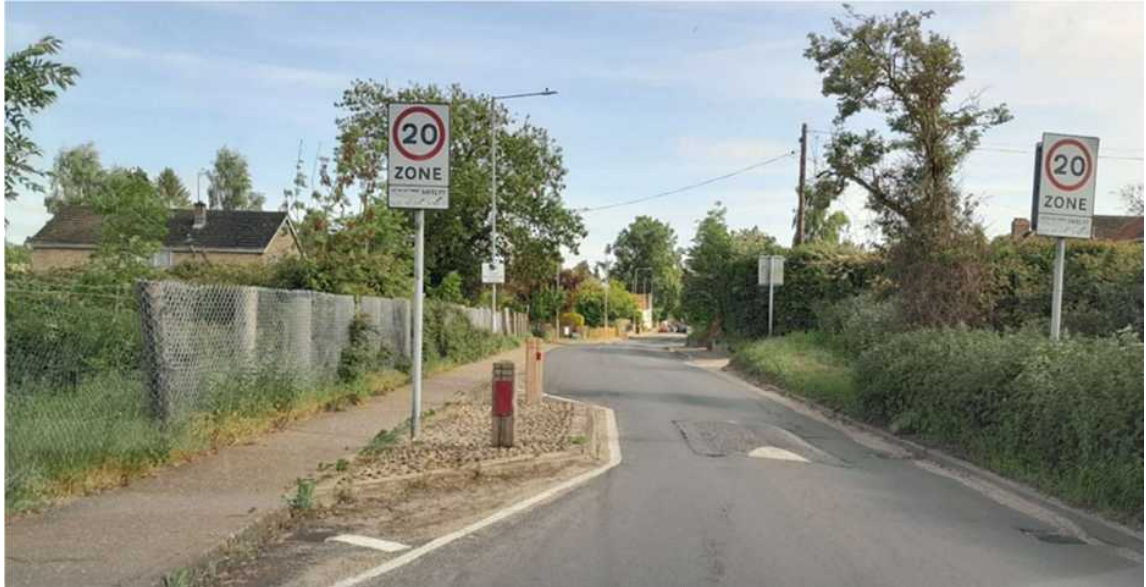
Figure 2-8 Traffic Calming Features at West End, Costessey
