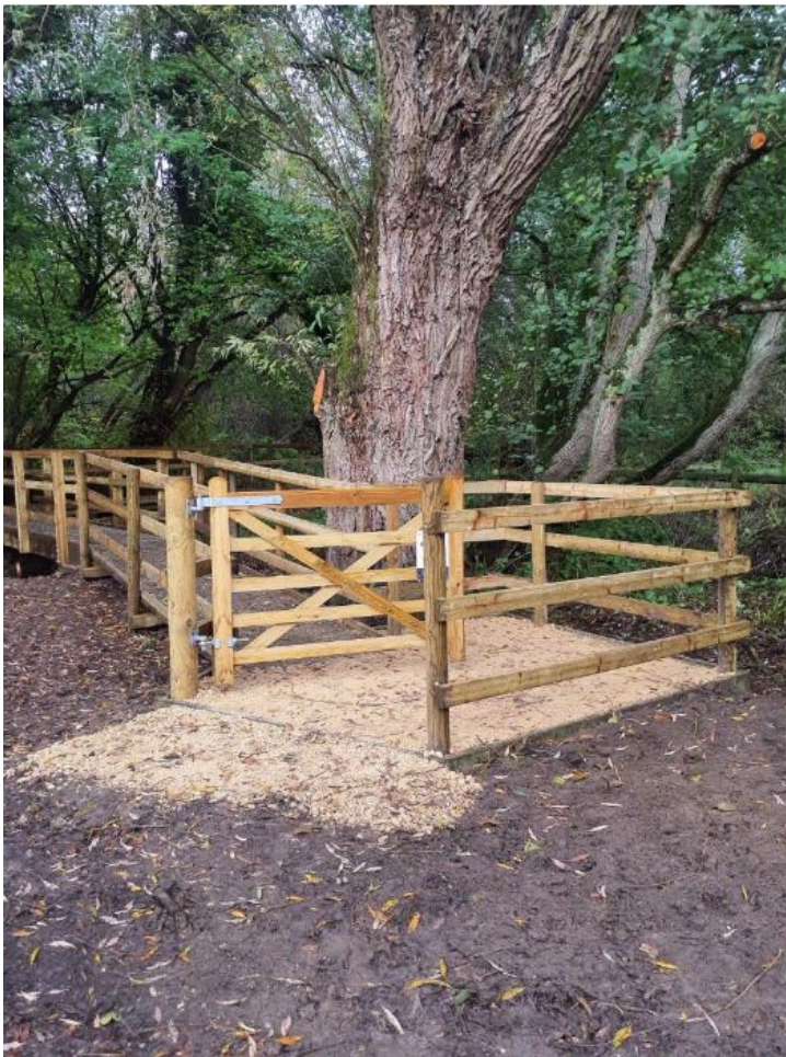
New kissing gate (footprint increased to accommodate build around mature tree)
