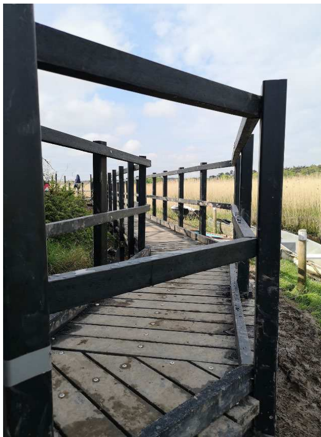
Image of the recycled plastic boardwalk construction at Cley next the sea.
