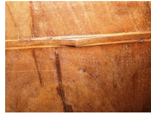
Close up showing damage to veneer
