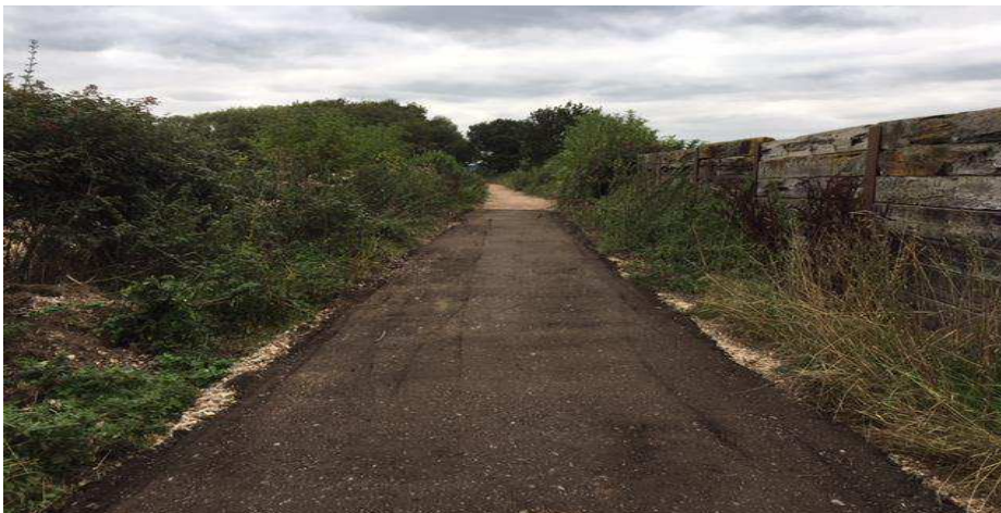
Naiden's Lane afterwards – vegetation clearance, base layer laid, drainage installed and resurfaced throughout.
